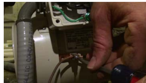
Figure 8. Make sure the ground bonding wire is securely fastened to the pump's bonding lug.
