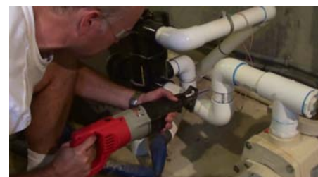
Figure 6. A reciprocating saw often works well to cut PVC pipe during the installation process.
