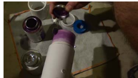
Figure 7. Thread sealant or pipe glue will help ensure fittings remain connected and leak-free.
