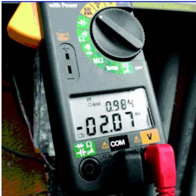
Figure 4. The RMS kilowatt meter can quickly and easily determine the pool pump's electrical consumption rate.
