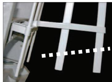
6. Trim bottom of barrier pickets if required as not to damage pool liner. Leave space between pickets and liner (6" maximum).
